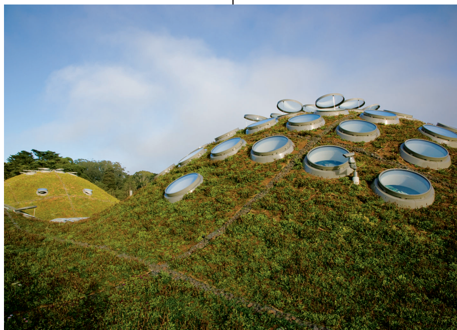
Coming soon, roof-top farming. Above, a two-acre green, “living” roof spans 12 buildings at the California Academy of Sciences.
