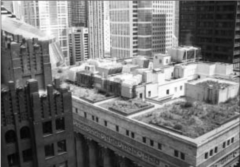
Figure 4. Green roof on Chicago City Hall
