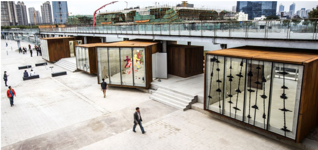
Image: Shanghai West Bund Biennial Pavilions (Source: Schmidt Hammer Lassen Architects)
