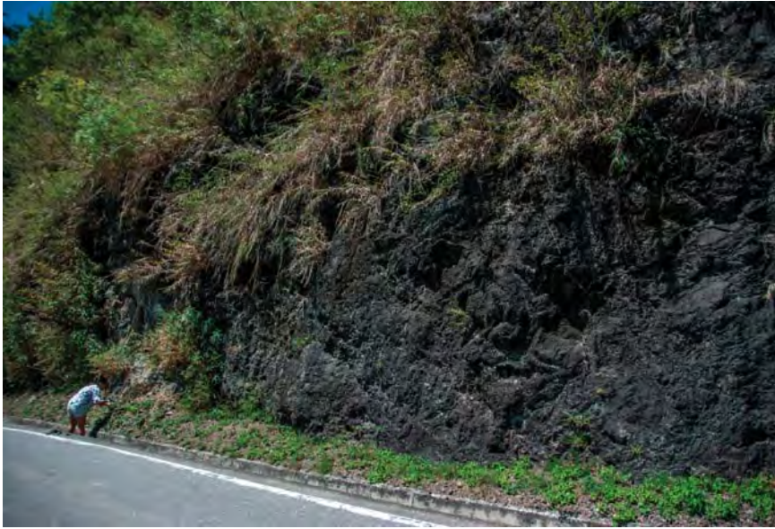
The roadcut by the Fanshuliao bridge.
